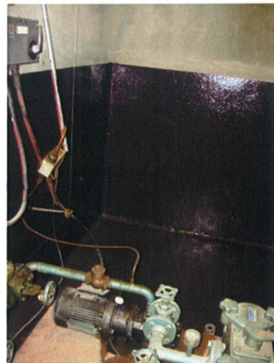
Deutschbank London – Diesel storage tank coating - internal
